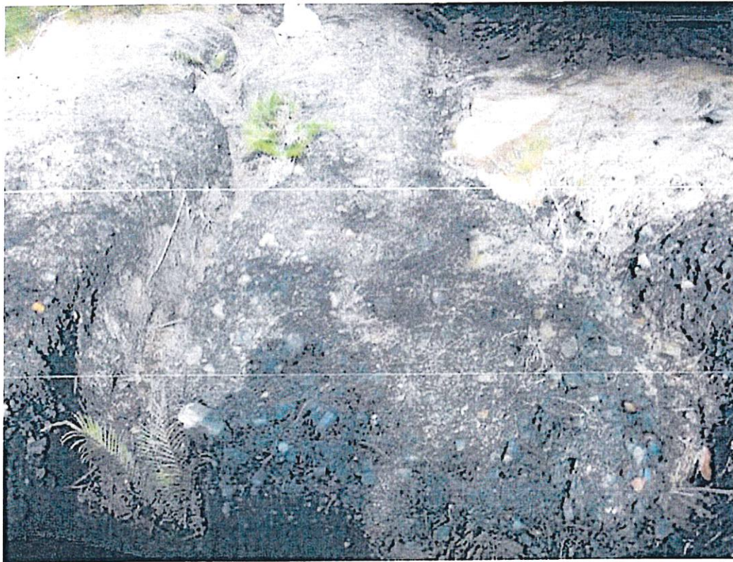
Figure 14- Close up picture of erosion pathway along the road shoulder, where coalwash was used.
