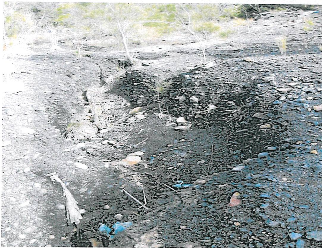
Figure 13- Gully erosion within the coal wash layer used for road construction on the road
