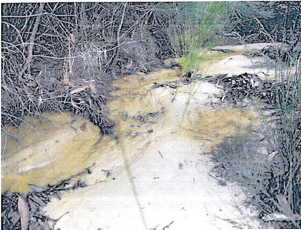
Figure 14- Close up picture of erosion pathway along the road shoulder, where coalwash was used.
